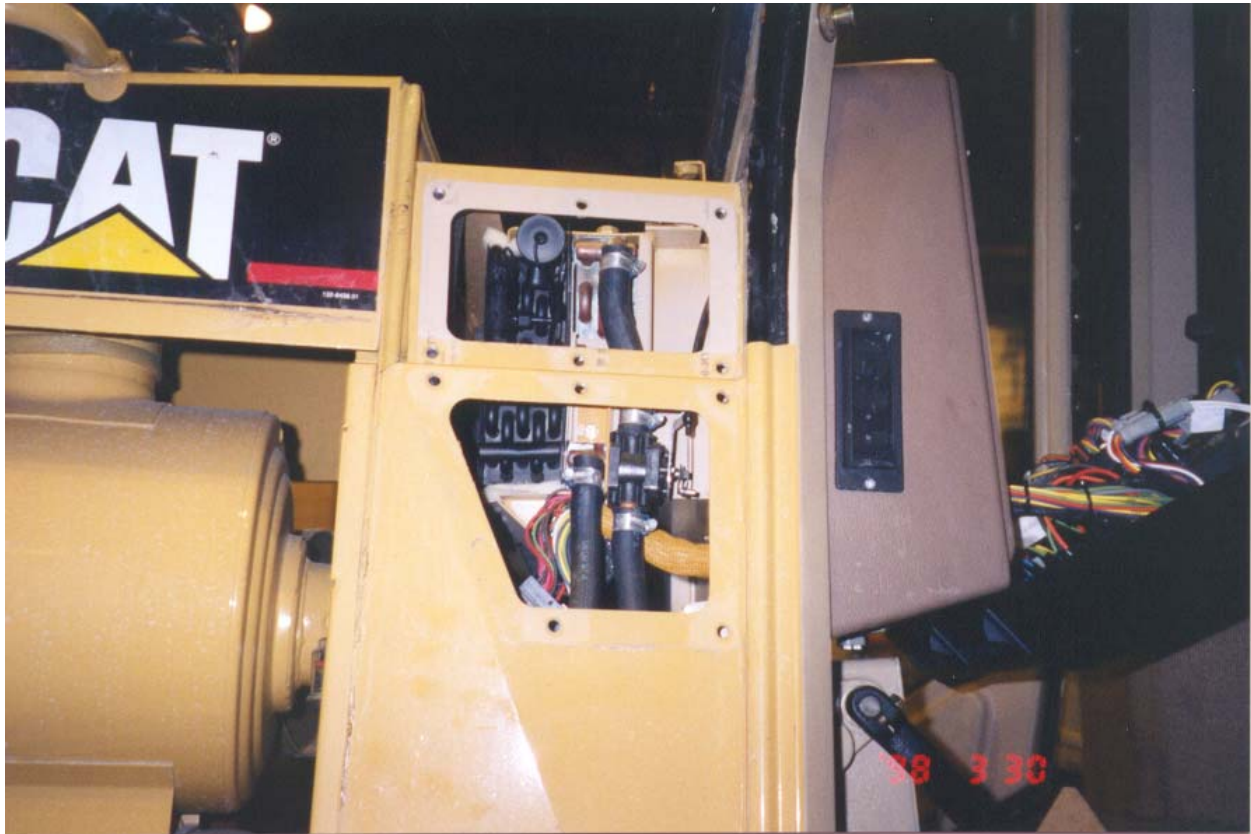
Evaporator in place alongside heater coil.
