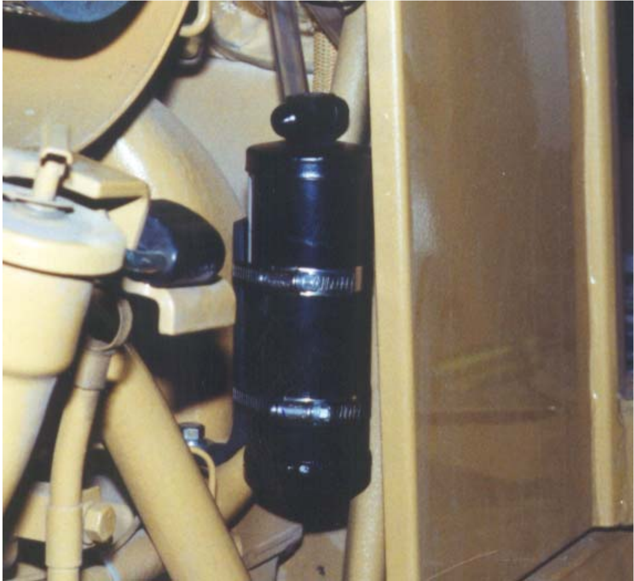
Drier in place.
